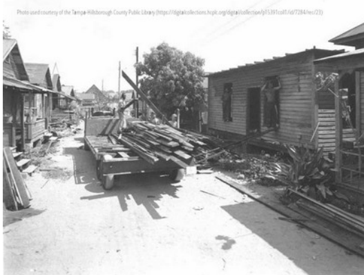
Figure 3. "The Scrub," in the process of being cleared (1952).
