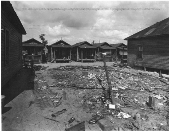
Figure 4. A lot in "the Scrub," after clearance for urban renewal (1952).
